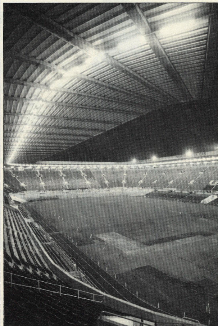
The slope of the seating gives variable mounting heights, and these had to be taken into account when planning the installation.
